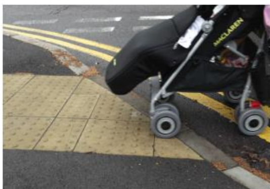
Dropped kerb with tactile paving
